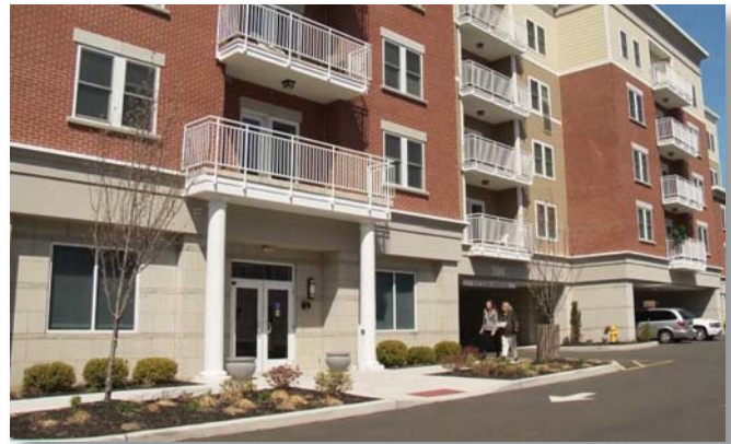
Marshall Commons senior affordable housing in Stamford's South End.
